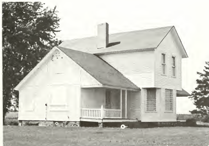
Partially restored locktender's house at Lock 19.
